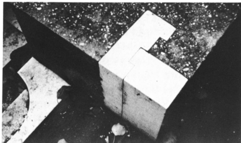
6 Palazzo Querini Stampalia; Venice, 1961-63. Garden corner detail. Concrete and white marble.
