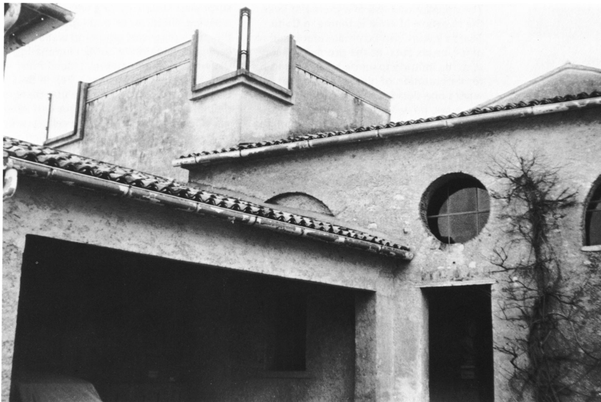
24 Gipsoteca Canoviana in Possagno, 1956-57. Window detail.
